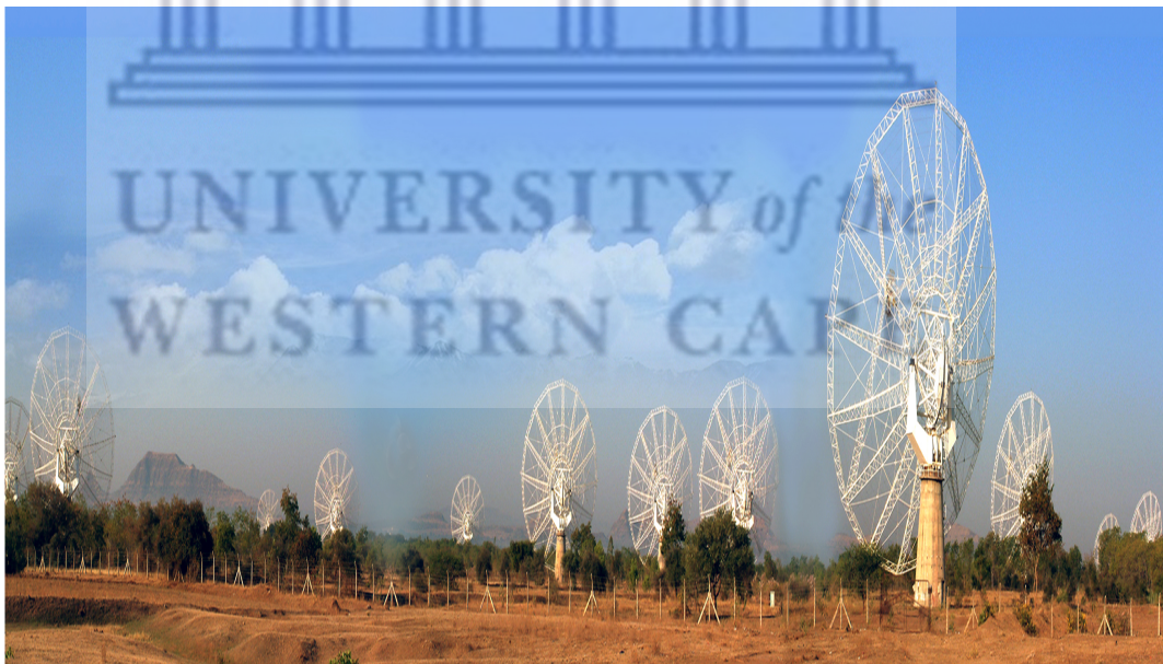
Figure 2: GMRT dish antennas in Pune, India. They cover a baseline distance of 25 km. Image courtesy of https://www.skatelescope.org/news/indias-gmrt-telescope-becomes-ska-pathfinder/ .
