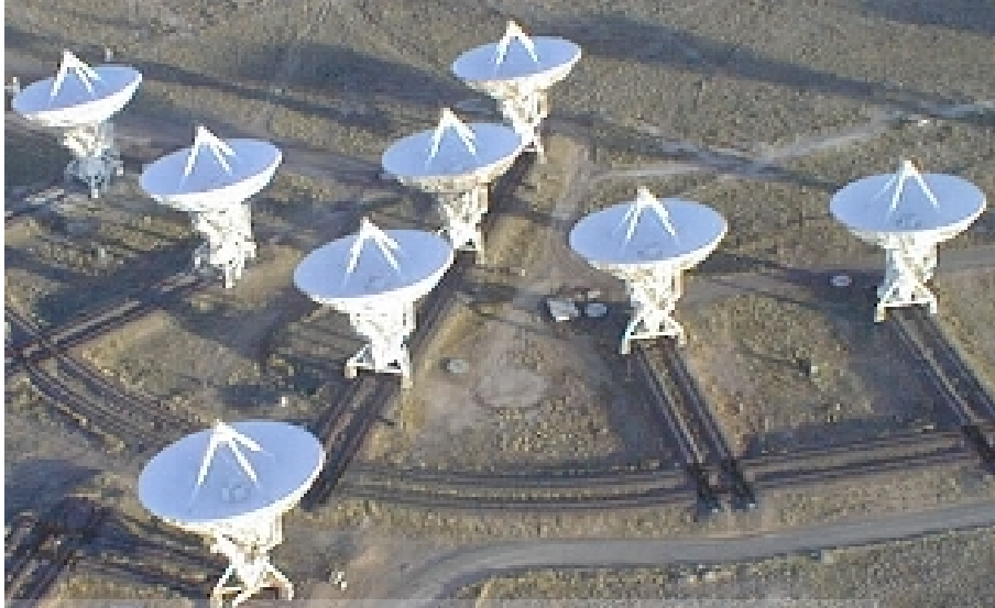
Figure 1: Image of a few radio antennae (dishes) of the Jansky Very Large Array in Plains of San Agustin, New Mexico. The rail tracks on the ground are used to control the baseline (resolution) of the survey. Image courtesy of http://www.vla.nrao.edu/
