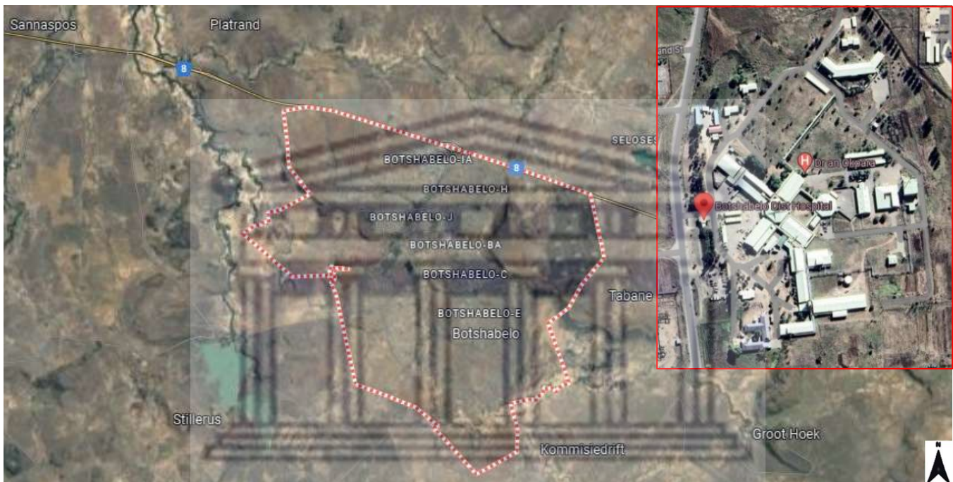
Figure 1: Locality of Botshabelo Township and BDH (Source: Google Earth, 2023)
