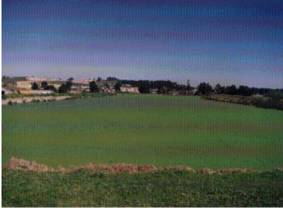
V. Sedimentation pond (Activated sludge is separated from the wastewater)
