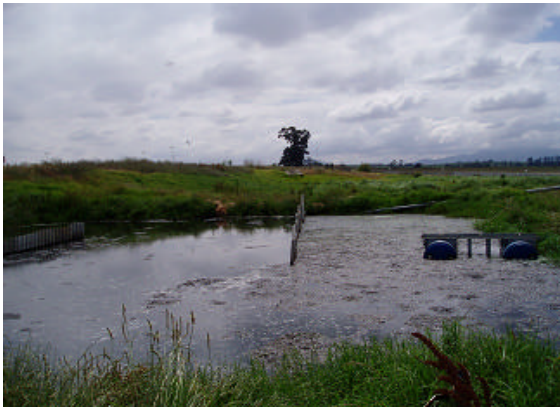
VII. Chlorination pond (Killing off the harmful bacteria)
