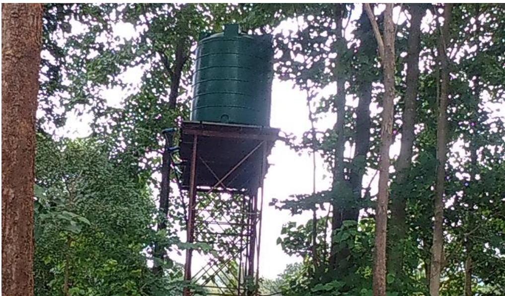
Figure 3: One of the water tanks at the studied school
