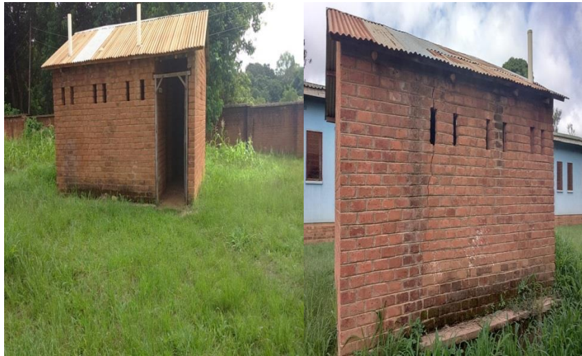
Figure 4: Pit latrine located behind Form 1 learners' hostel
