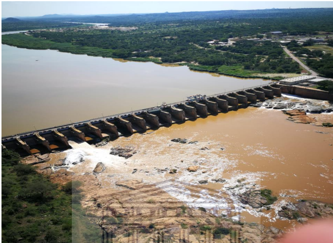
Figure 3.3: The barrage for Phalaborwa WTW
