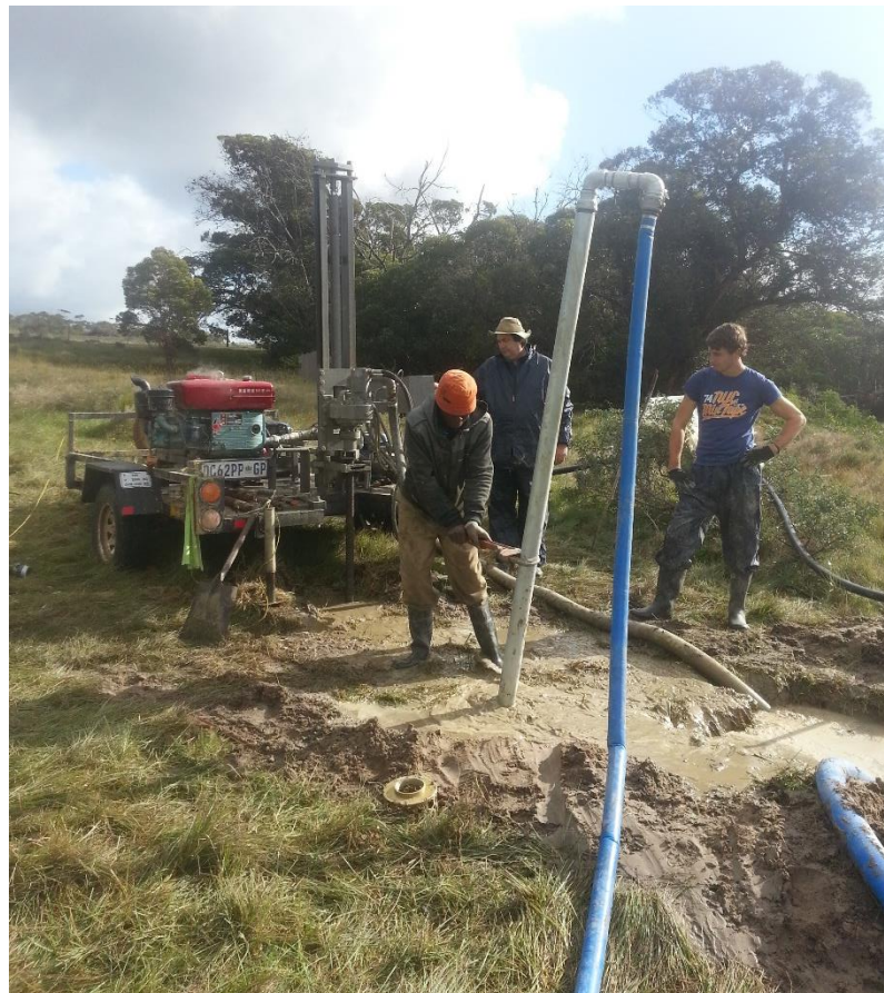
Figure 24: Mud-Rotary drilling and hydraulic jetting method
