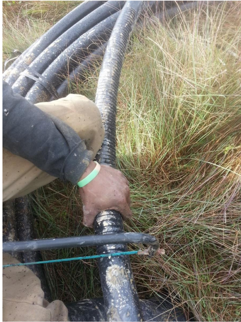
UNIVERSITY of the WESTERN CAPE Figure 27: Piezometer slots
