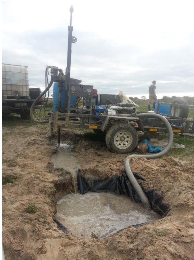
Figure 22: Mud-Rotary drilling
