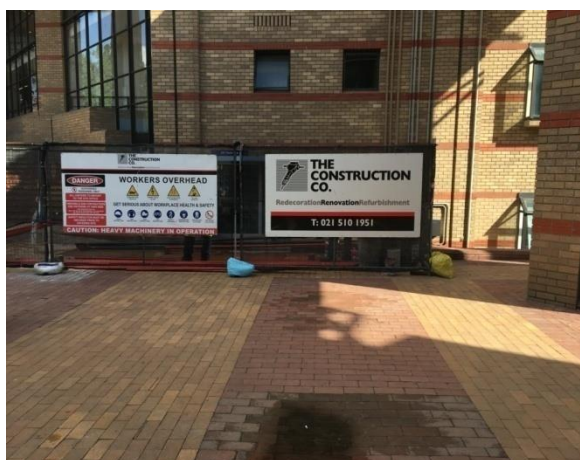
Figure 4.18: UWC library renovations 2019
