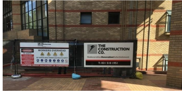
Figure 4.18: UWC library renovations
