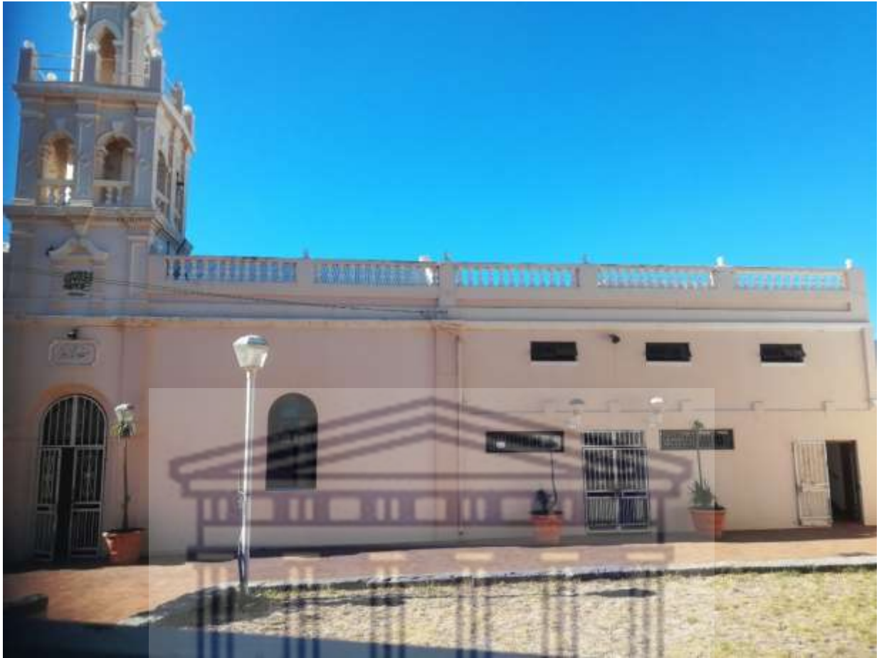
Figure 5. 10 Al-Azhar Mosque in Cape Town, with three unlabelled entrances. Main entrance on the far left is for men. Entrance at the far right is where I entered to go to the upstairs women's area. The Arabic script above the main door is the name of the mosque.
