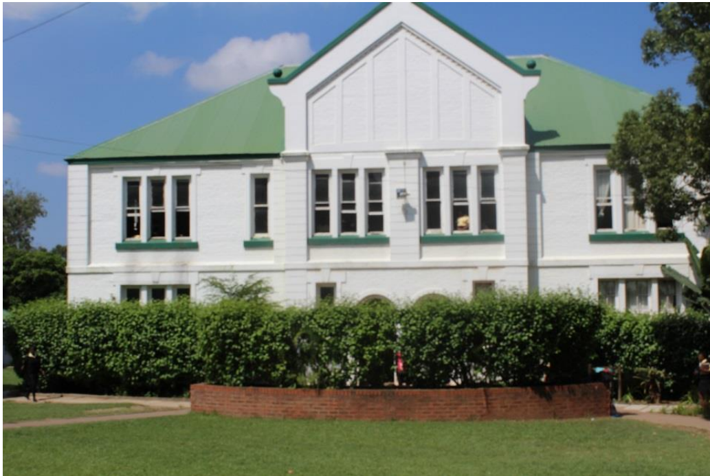
Figure 35. The last structure built when Edwards was still alive was originally used for sewing classes.
