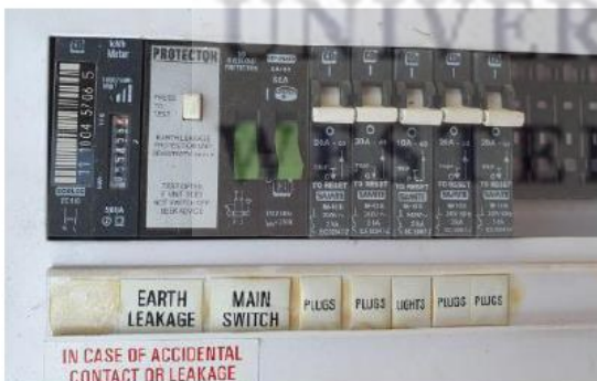
Diagram 3 : Current Distribution Board with all circuit breakers OFF.
