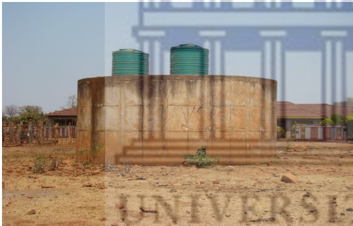
Figure 5. 15 Village reservoir; a booster pump is sufficient to fill tanks; however, no diesel is supplied by Municipality to operate it.
