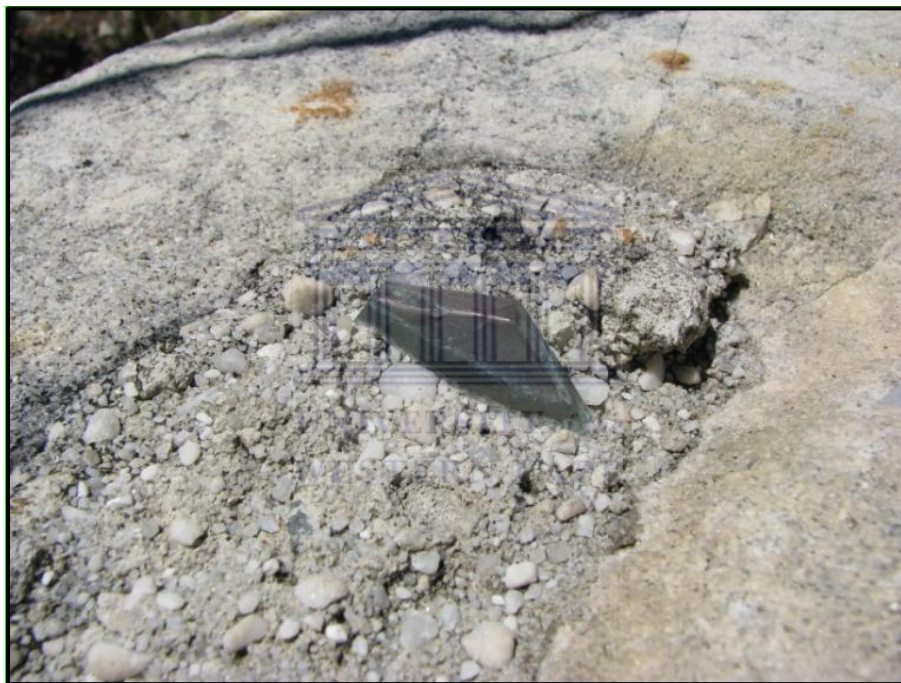
Figure 12. The original copper markers used to mark the permanent plots were cemented into the sandstone rock and mixed with sandstone grit. Note the ‘cement’ erosion line on the marker, where approximately 2 – 3 mm has eroded. This shows that that considerable erosion and leaching of cement has taken place over the 33-year period. Cement and concrete occurs in the form of the path networks (both new and old) and very large amounts of debris on the Western Table.
