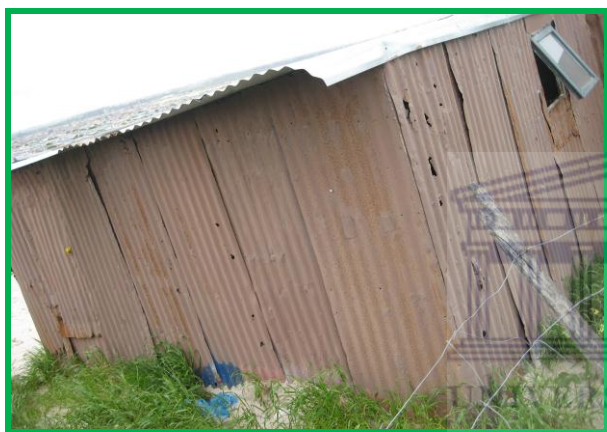
Figure 11: A small and high window, as an emergency exit.
