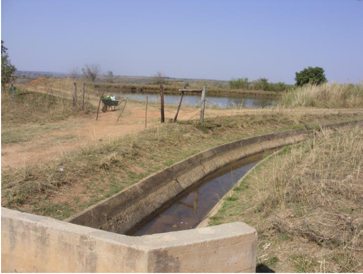
Figure 9: Feeder canal drawing water from a reservoir to farmers' fields at New Forest irrigation
