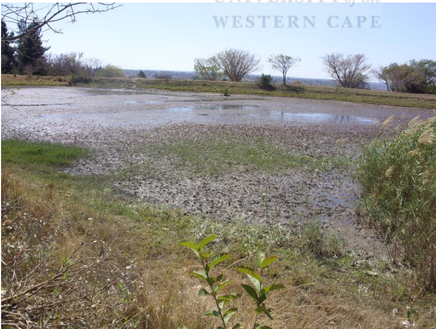
Figure 12: Reservoir that has been silted and overgrown with grass and shrubs
