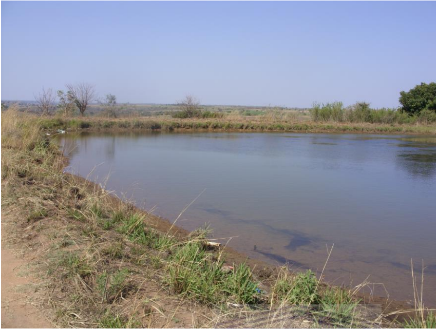
Figure 11: One of the reservoirs storing water for the irrigators
