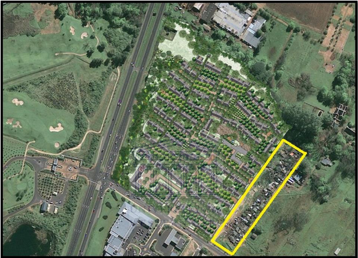
Figure 3.3: The image above shows an aerial image of La Clemence Retirement Village with the R44 main road on the western boundary, Webervallei road (Jamestown main road) in the south and the informal settlement demarcated by the yellow block on the eastern boundary.
