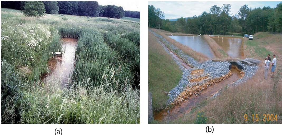
Figure 2.2.1: Typical passive biological (a) and chemical (b) treatment of mine water systems (INAP, 2012).
