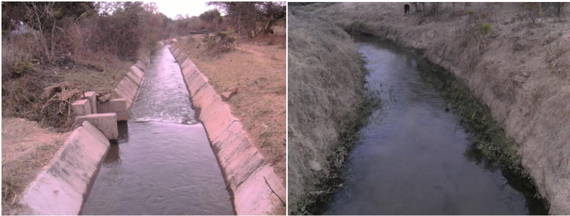
Figure 5: The Lined and the Unlined Sections of the Main Canal
