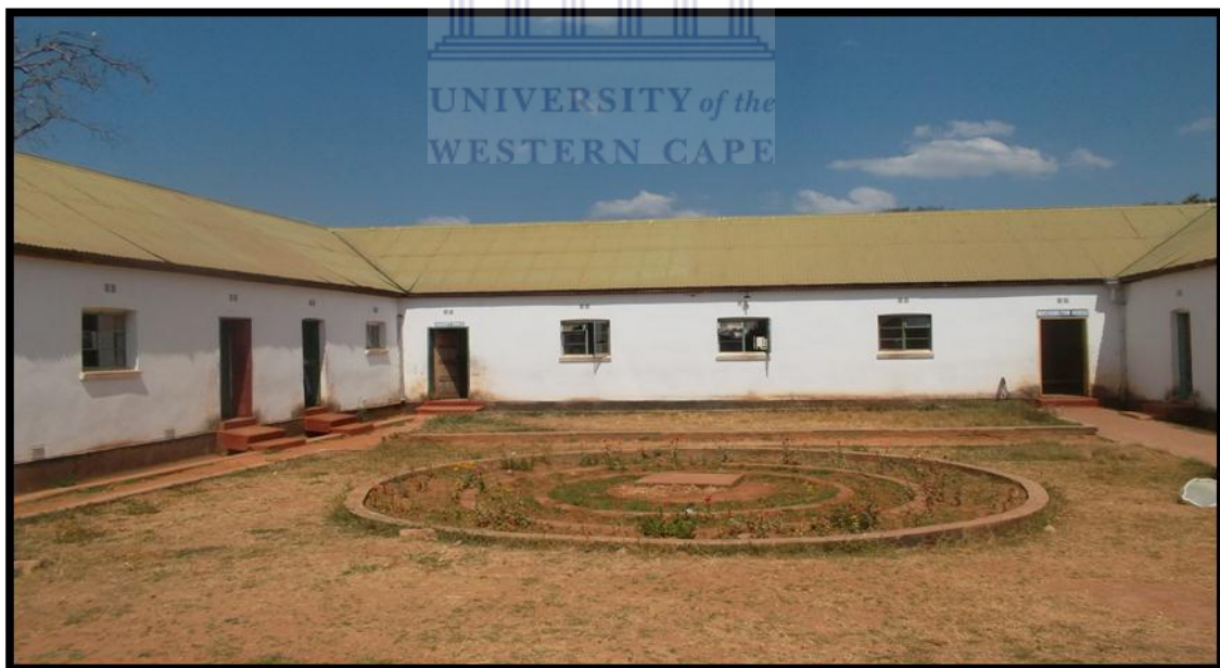
Figure 15: The old jail constructed in 1891 which is now being used as a dormitory by female students at the mission school. (Photo by N. Chipangura)
