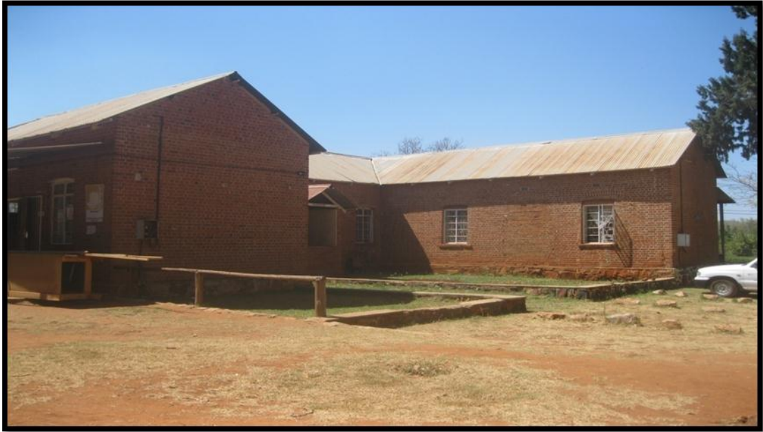
Figure 12: A full view of the building that was constructed in 1891 and now used as an administrative block by the mission school. (Photo by N. Chipangura)
