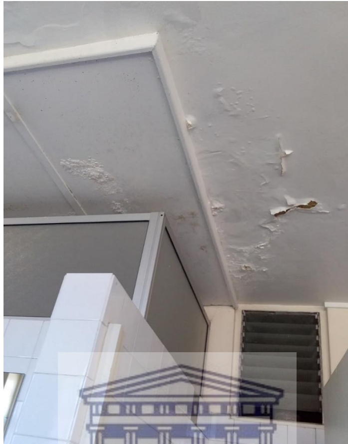
Figure 6.16 . Residence bathroom ceiling
