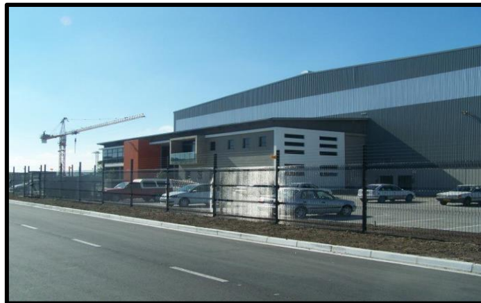
Figure 7.2: GLS trolley repair unit, Pick n Pay. Philippi.
