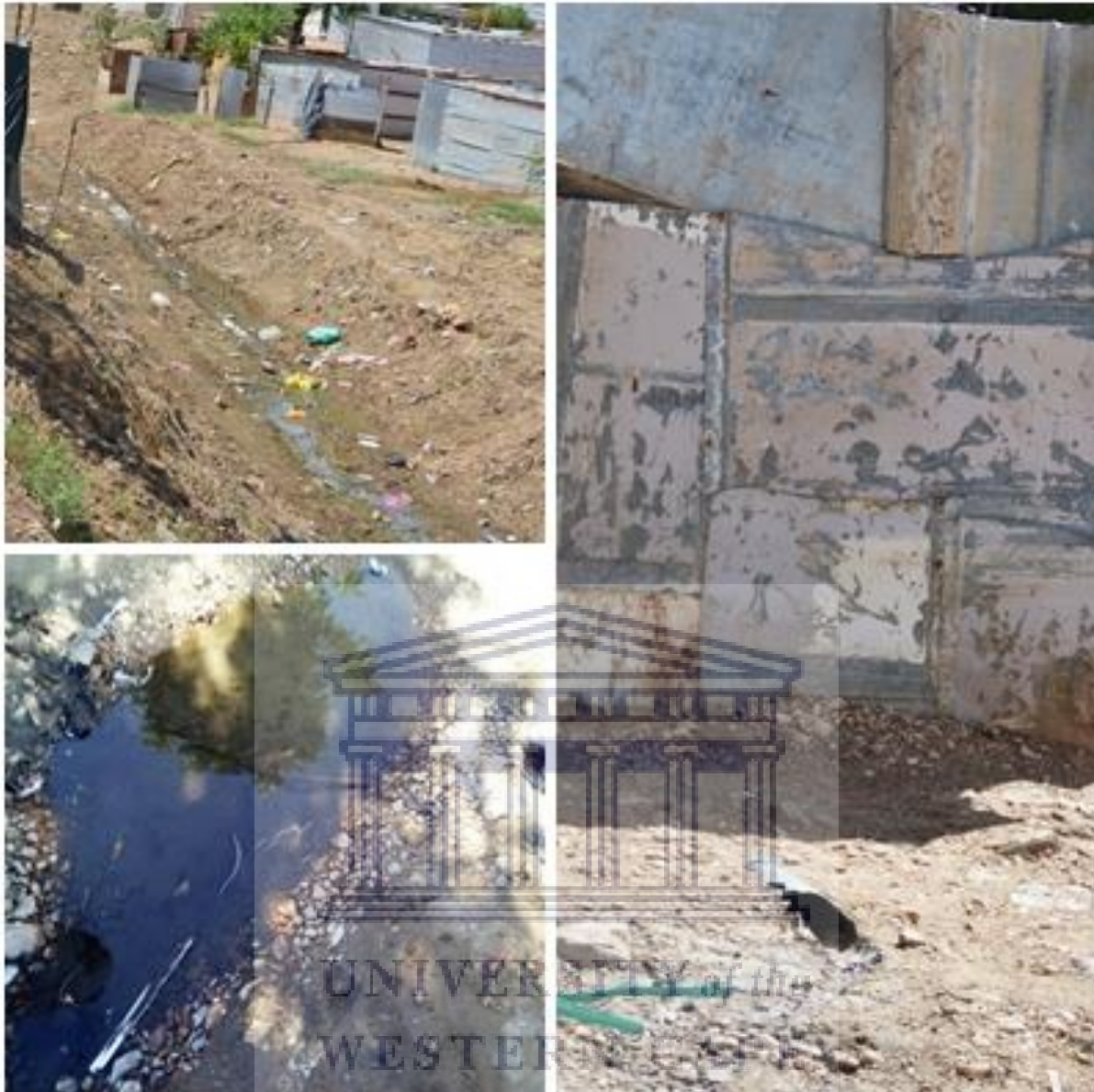
Figure 5.11 A photo of the Greywater spillage and lack of sewerage systems taken by the author in Havana informal urban settlements, Windhoek. February 10, 2018
