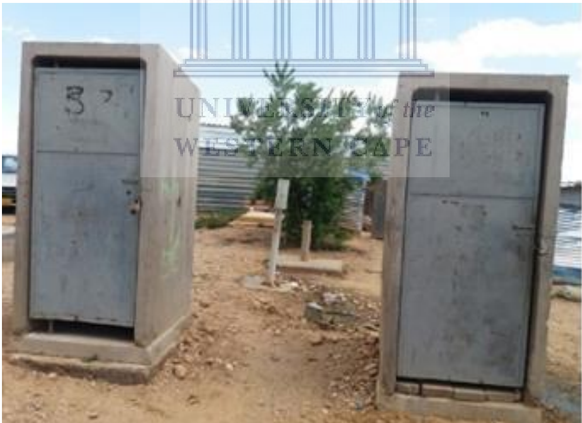
Figure 5.7: A photo of the Communal toilets built by the City of Windhoek taken by the author in Havana informal urban settlements, Windhoek. January 27, 2018
