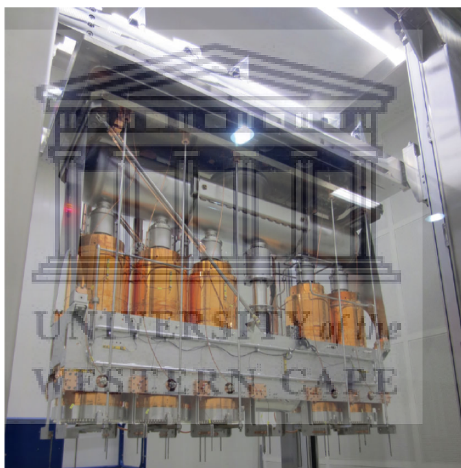
FIGURE 3.7: One of the cryomodules being installed in the ISOLDE hall. [7]
