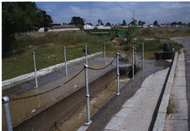
I. Input (Raw wastewater flows into the Scottsdale WWTW)
