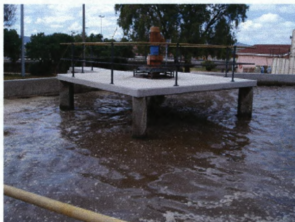
IV. Anoxic pond (Removal of nitrogen by microorganisms to optimize the operation conditions)
