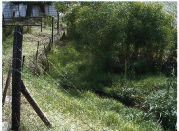
VIII. Outlet just outside WWTW (Final effluent discharges into the river)
