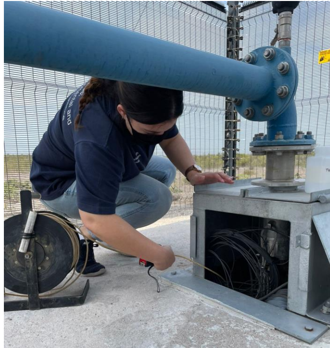
Figure 4-6: Measuring water levels at Langebaan Road wellfield using a dip meter
