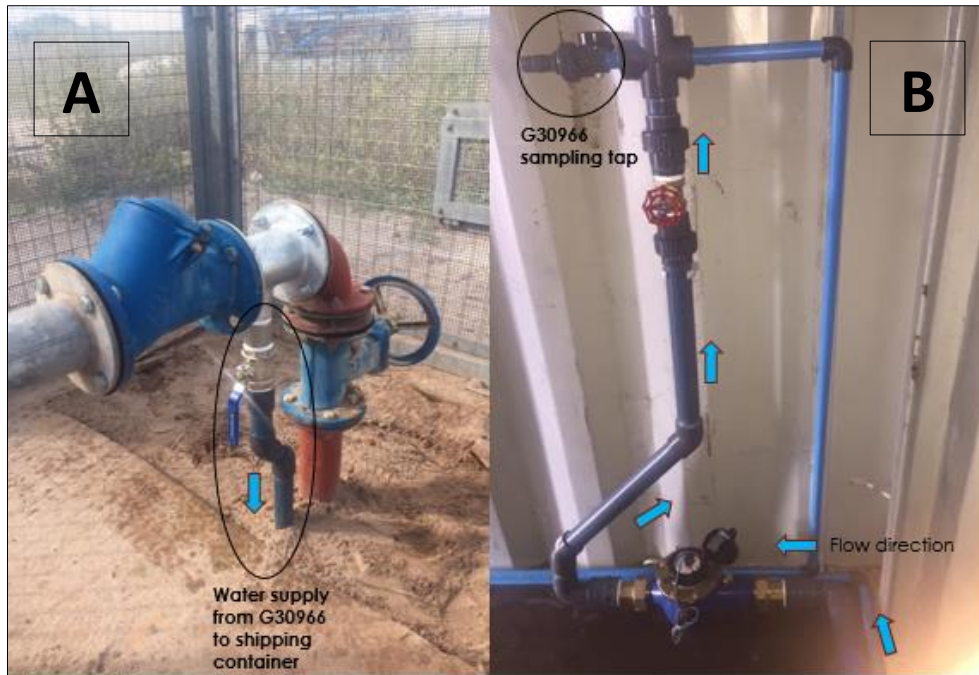
Figure 4.1: A. water supply and direction of the flow of groundwater abstracted from production borehole. B. flow direction of the groundwater into the shipping container from the production borehole.
