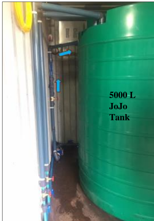
Figure 4.3: The flow direction of the groundwater extracted from production borehole (G30966) and into the 5000 L JoJo tank before dosed with ozone ( O_3 ) inside the shipping container at the study site, Atlantis.
