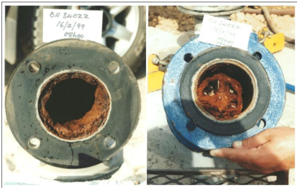
Figure 1.2: Iron-related borehole clogging experienced at the Atlantis Aquifer in the distribution pipeline (left) and flow meter at borehole (BH) 34022 in 1999 (Robey, 2014).
