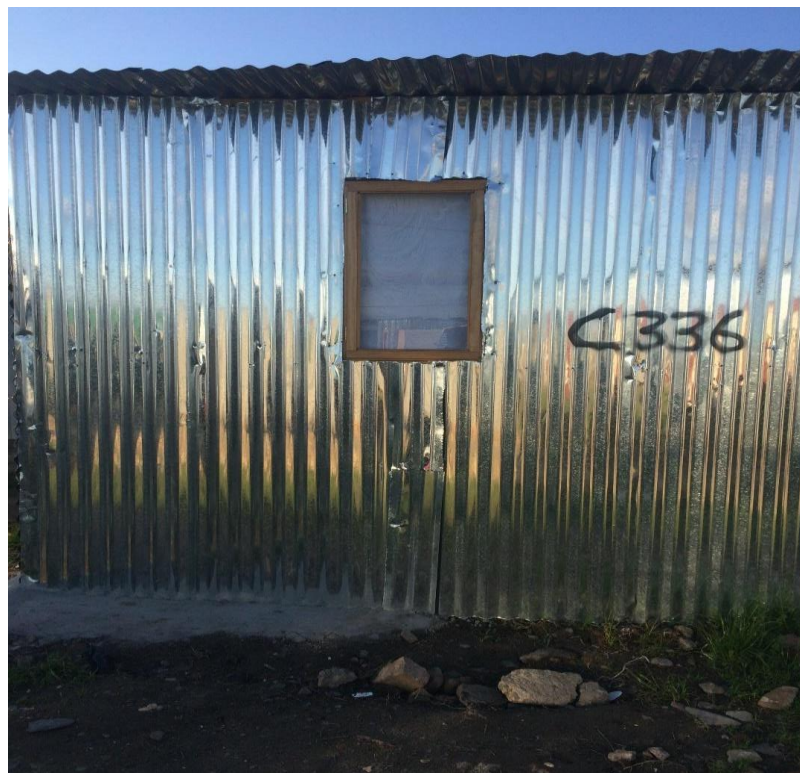
Figure 3: One of the houses marked by the residents, with a marking spray.
