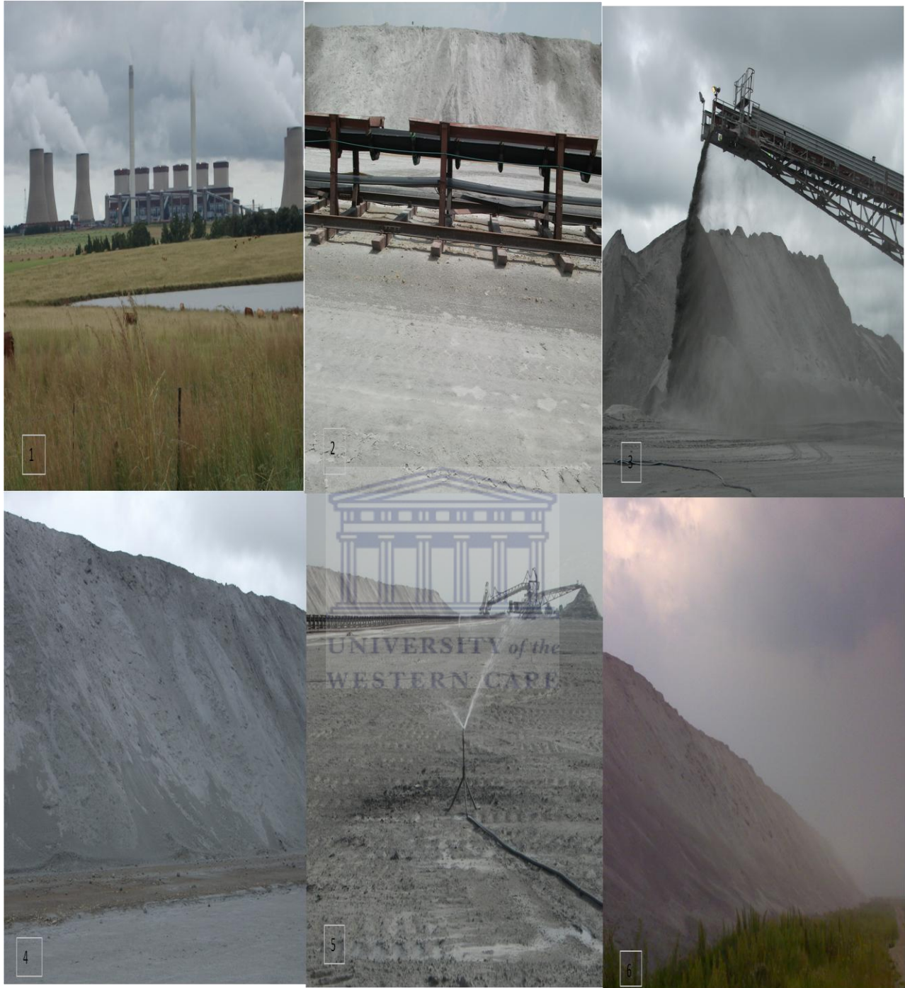
Photo 2.1. The photographic setting of the Tutuka ash dump showing ash deposition, brine irrigation, and the areal extend of the ash dump. Stage 1 is the power station where coal is burned while stage 2 the by product of burned coal ash transported via conveyer belt onto the ash dump and deposited as shown in Stage 3. The deposited ash is then compacted in the form of stacks before irrigating the ash for dust suppression as shown in stage 4 and 5. Stage 6 provides an idea on the extent on the ash dump in the North - South direction.
