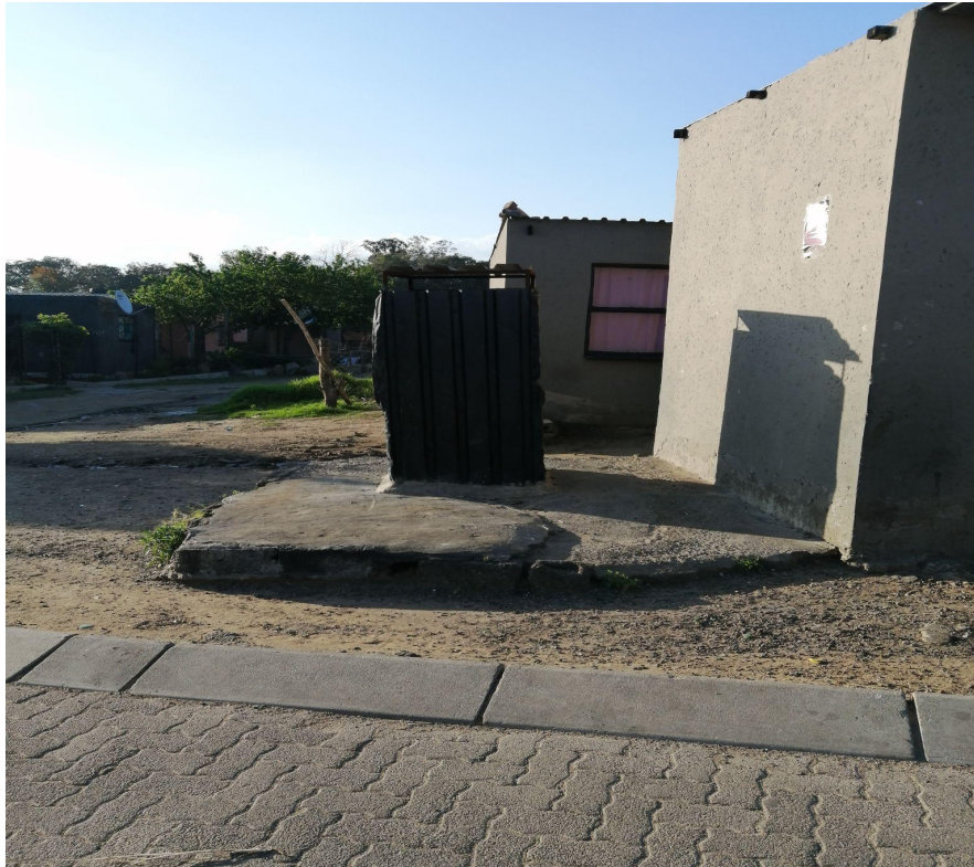
Figure 9: A pit toilet next to a home
