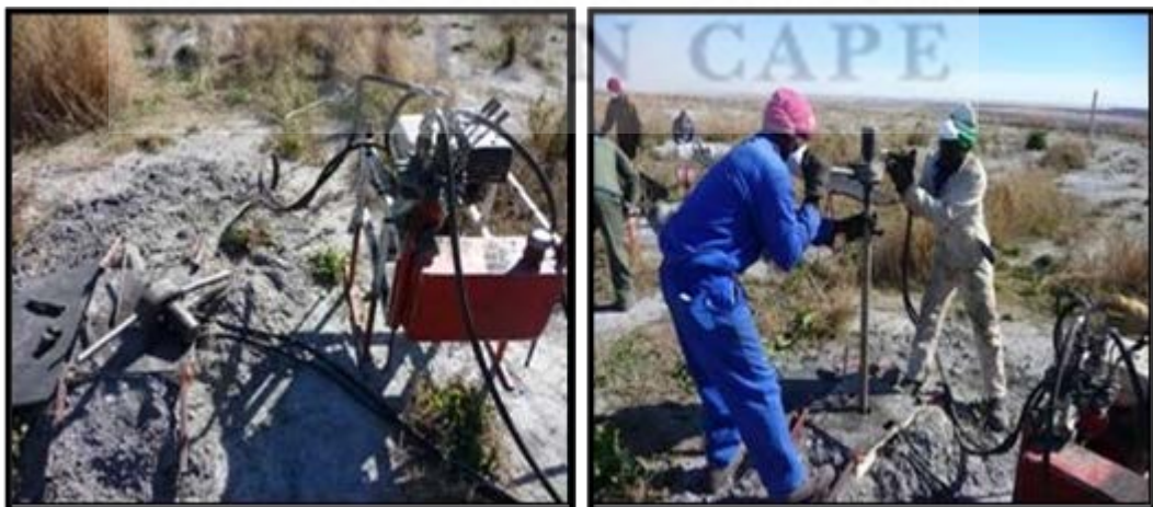
Figure 3.1: Drilling process at SASOL Secunda ash dam
