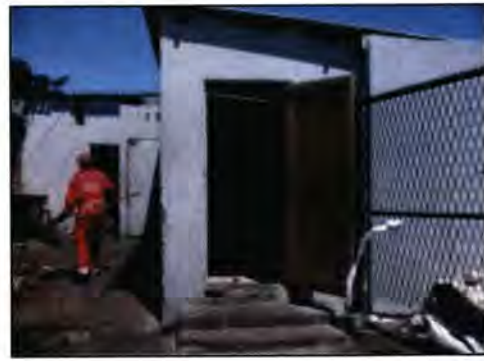
Plate 7.10 Concrete Enclosed Toilet
