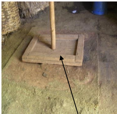
Fig 3: toilet with covering
