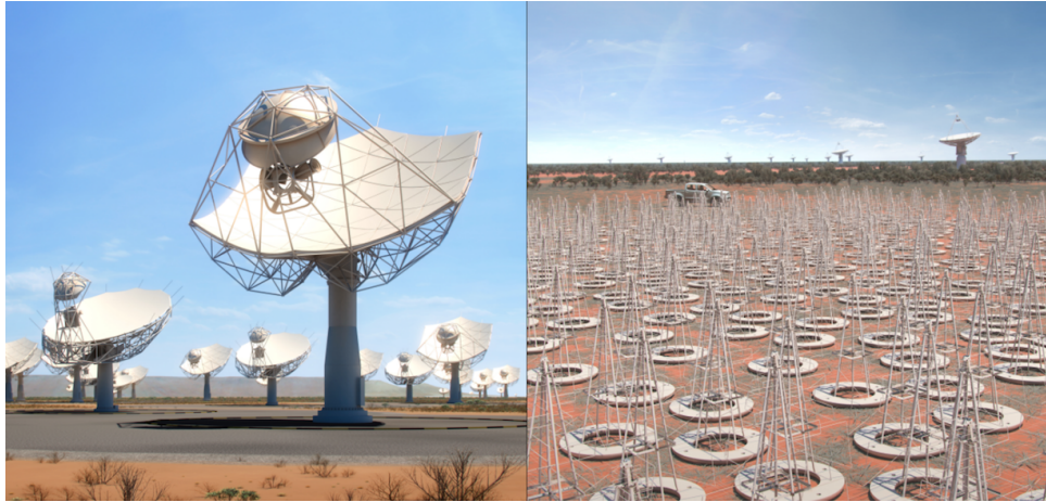
FIGURE 1.3: An artist rendition of the SKA array. Left: The SKA-MID instrument that will carry out mid-frequency observations. It will be located in South Africa. Right: The SKA-LOW instrument that will carry out low-frequency observations. It will be located in Australia.
