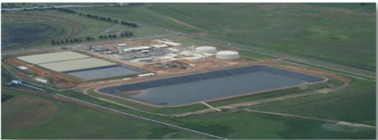
Figure 5: The eMalahleni Water Reclamation Plant. Adapted from (Petrik et al. , 2015).
