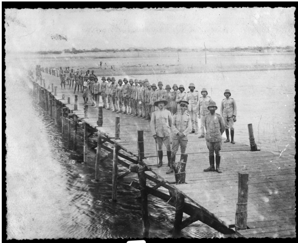
Figure 5. On the trestle bridge over the Rovuma River. PT AHM-FE-110-B7-GR-1.10.
