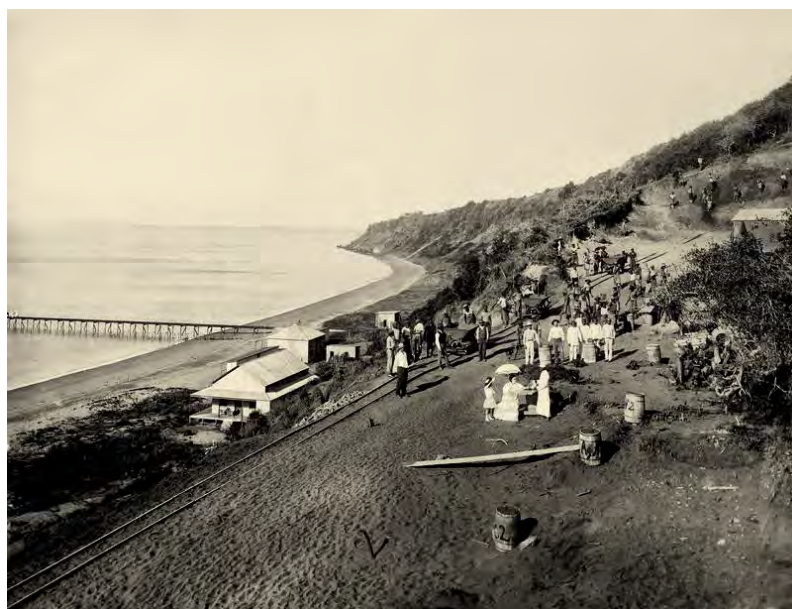
Figure 2. Polana beach. Caracol road in an early stage of its construction.
