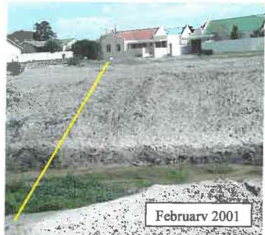
Plate 5.1: Cross-section 2.3 on the right bank before and after the channelisation. Flow was from the right to the left.
