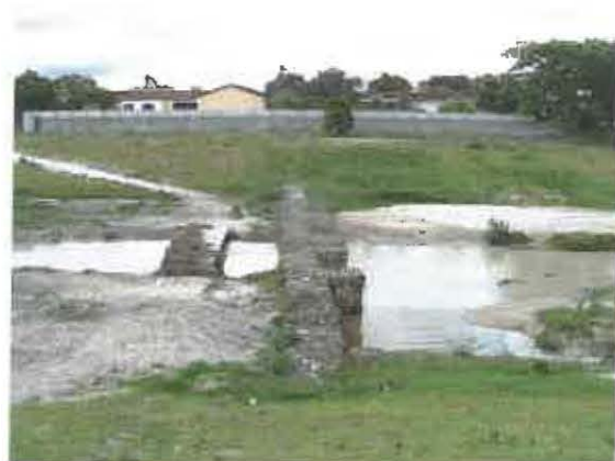
Plate 5.6: Sediment deposited on the floodplain area, within the channel and behind the gabion weir in Site 3 after the floods. The vegetation on the floodplain areas was completely buried under the sediment.
