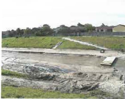
Plate 5.6: Sediment deposited on the floodplain area, within the channel and behind the gabion weir in Site 3 after the floods. The vegetation on the floodplain areas was completely buried under the sediment.
