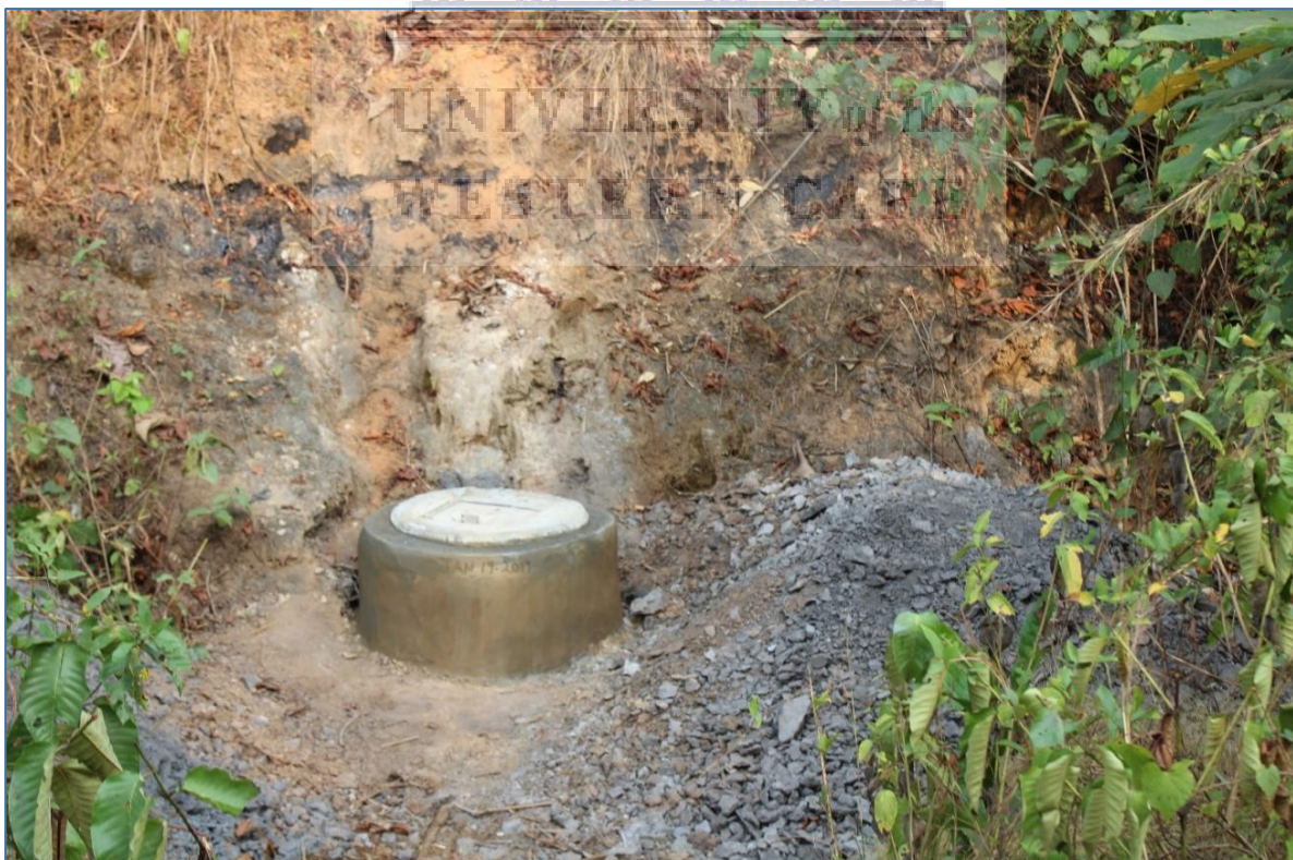
Figure 26: Field photograph showing wellhead after drilling and sample acquisition.
