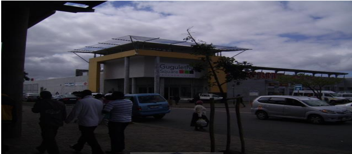
Figure 3 Gugulethu Square mall from outside
