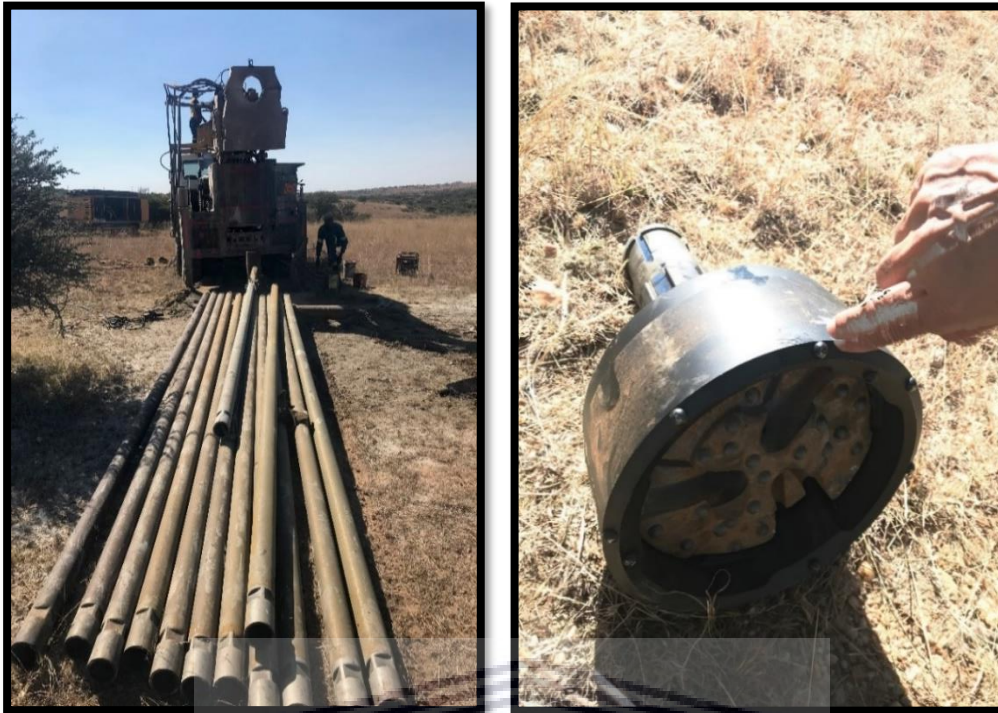
Figure 4.8 Steel rods and drilling bit
