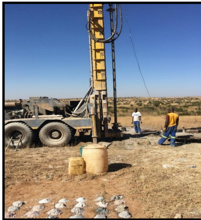
Figure 4.7 Air-rotary drilling on the Ga-Mamadila site
