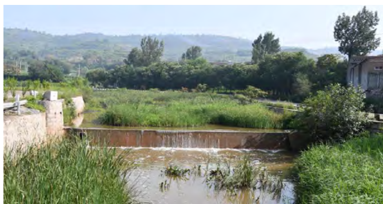
Figure 5-3 Overflow weir of Shandi River
