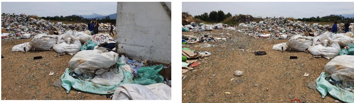
Figure 49: Newly allocated area on the Wellington landfill
