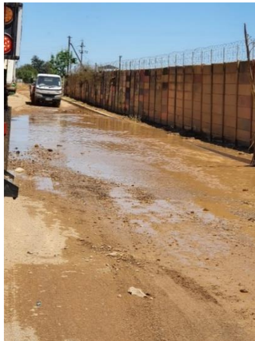
Figure 44: Road leading to the entrance of the landfill
