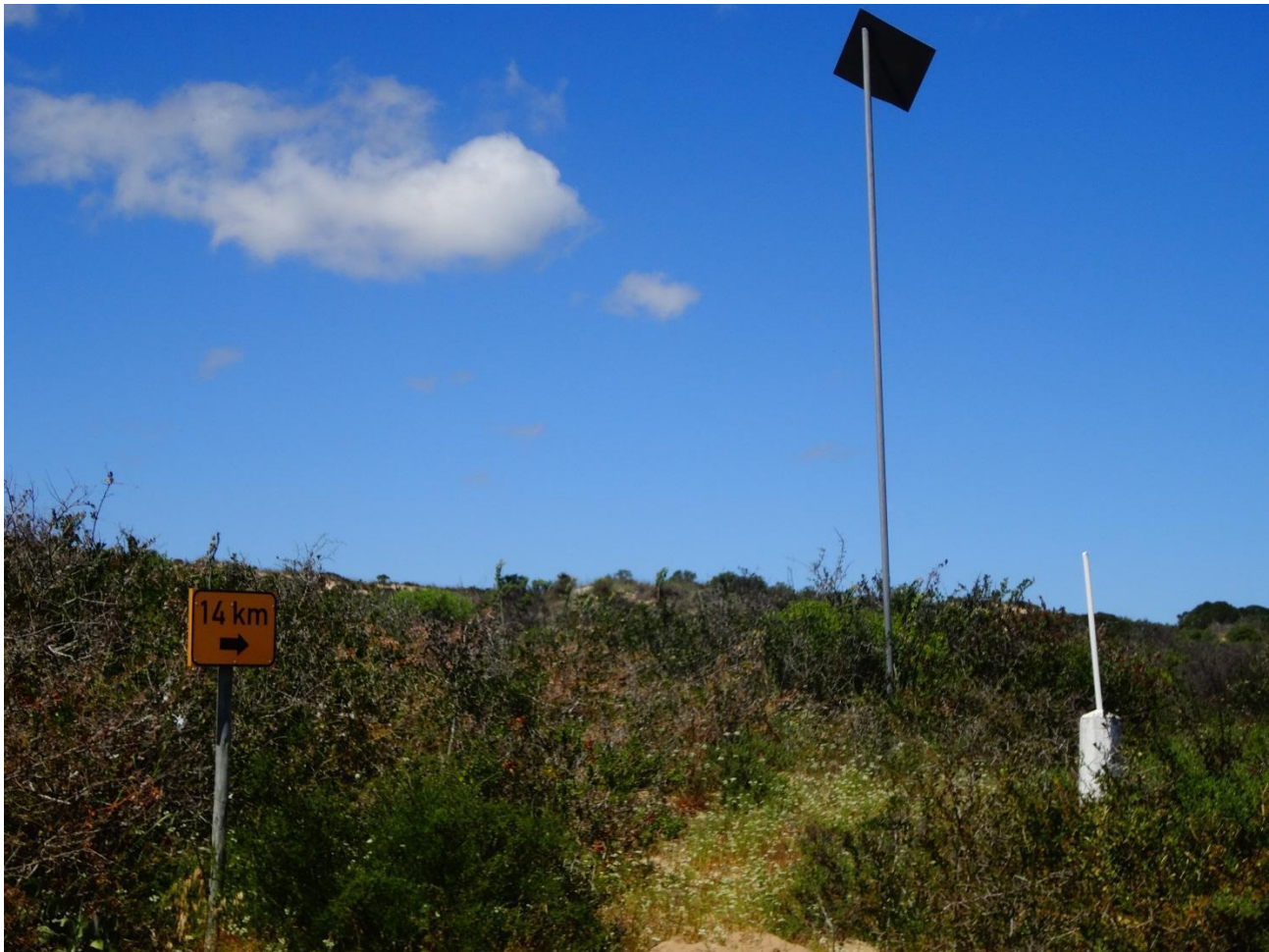
Figure 6.22: Location of the underground oil pipeline in the WCNP – indicated by the high mast
