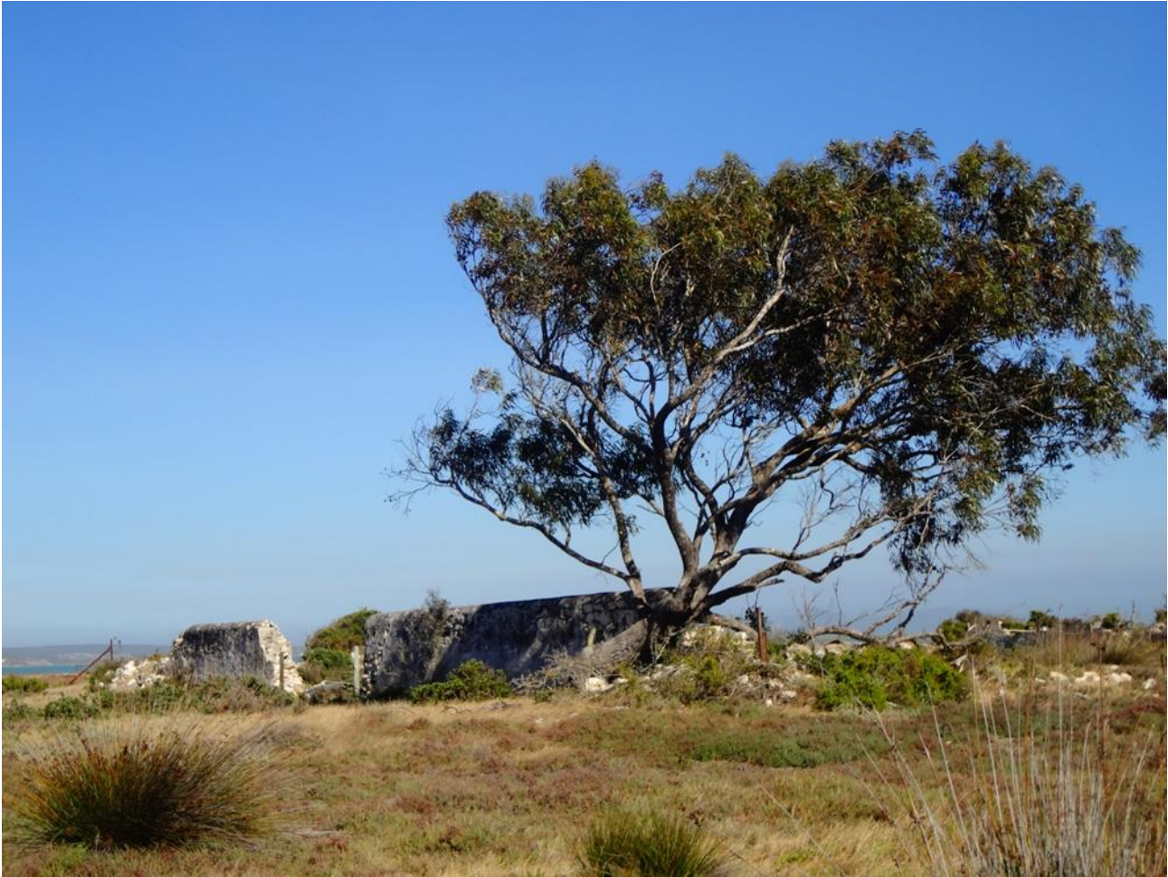
Figure 6.12: Ruins of the old abattoir that used to serve the farming communities that existed near Geelbek before the proclamation of the WCNP.
