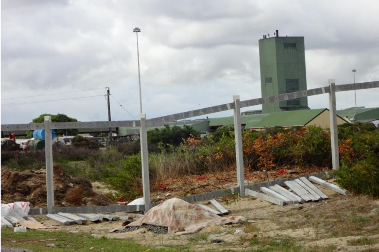
Figure 5.19: A new re-aligned boundary under construction in 2018 with concrete palisade fencing
