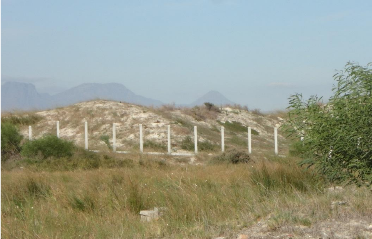
Figure 5.20: The incomplete fence between sparsely vegetated dunes and the area west of the Green Park informal settlement
