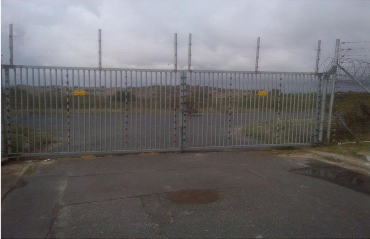
Figure 5.22: Electrified gate and fence
