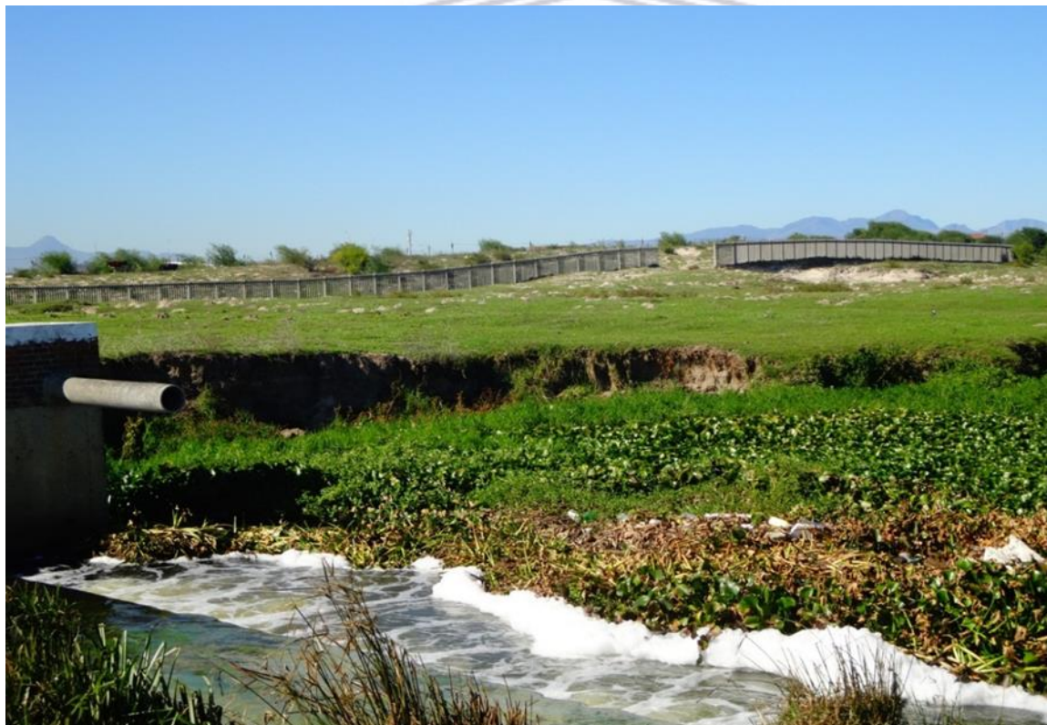
Figure 5.5: Fluid waste disposed in the Kuils River on the eastern boundary of DNR
