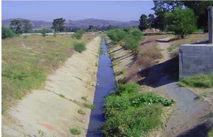
Figure 6. The channelized De Novo tributary (site 6.1)
