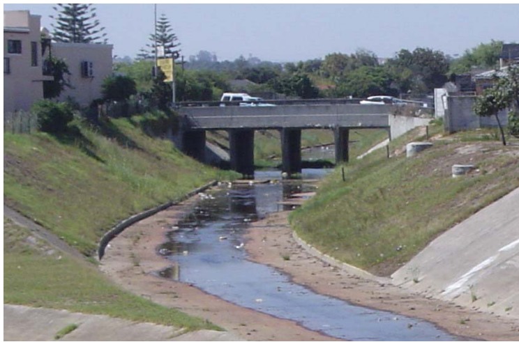
Figure 7. The channelized lower end of the Bottelary River
