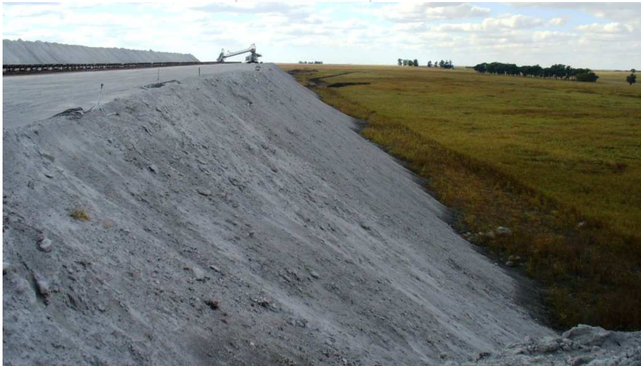
Figure 4.1. Horizontally stacked dry disposed ash in Tutuka ash dump site.
