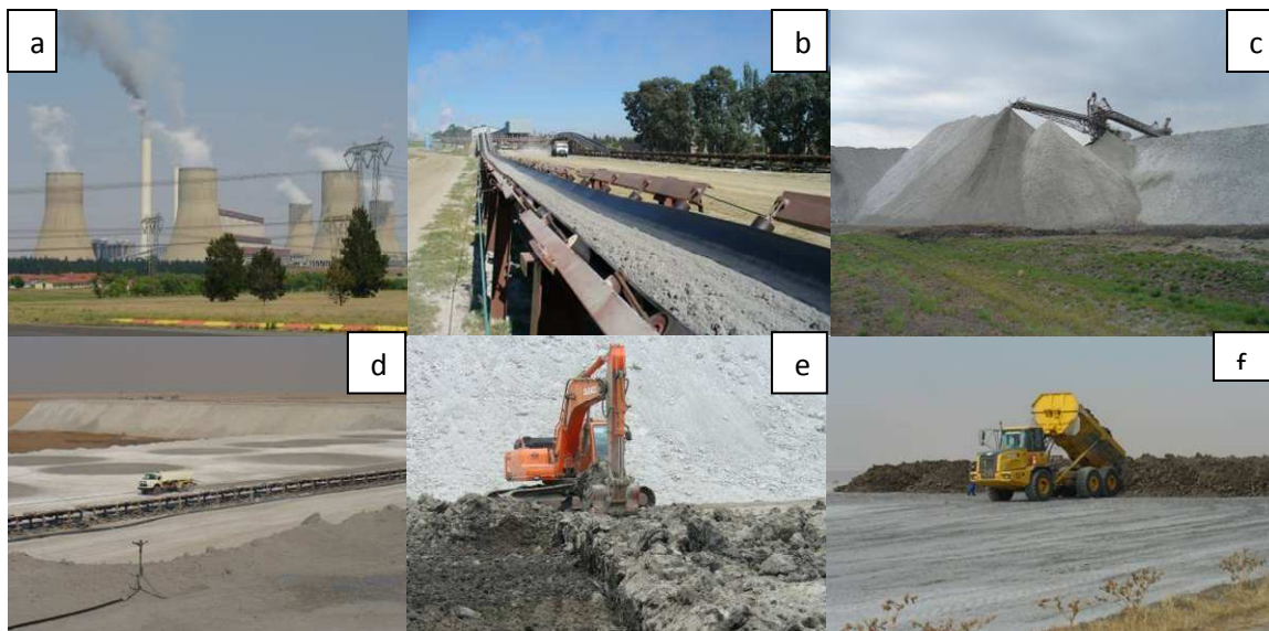
Figure 3.3. Photograph of dry ash disposal system at Tutuka Power Station (After Petrik et al. , 2008).
