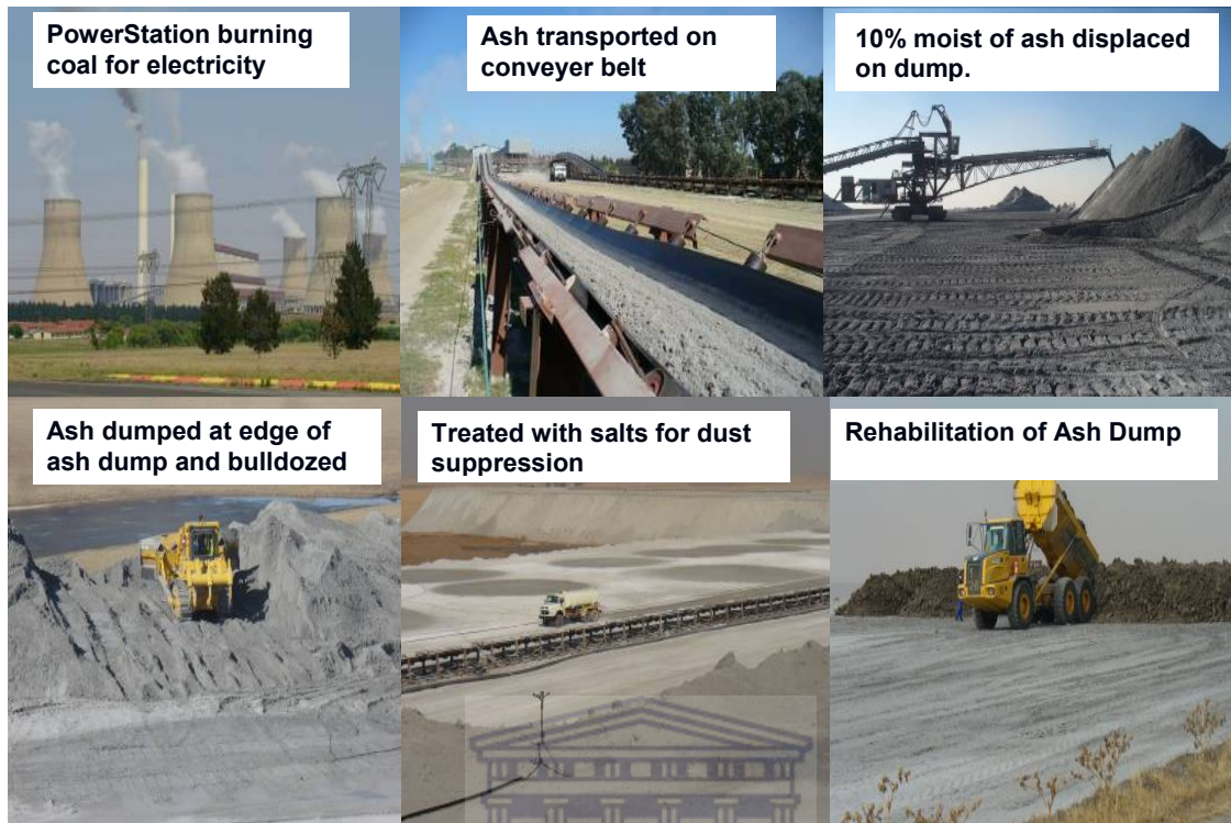
Figure 3.2 Ash dump system formation showing power station where coal is burned, the by product of burned coal ash transported via conveyer belt onto the ash dump, compacting the ash by compaction and suppressing the ash by irrigation and then irrigating the ash for dust suppression ,rehabilitation of ash dump.
