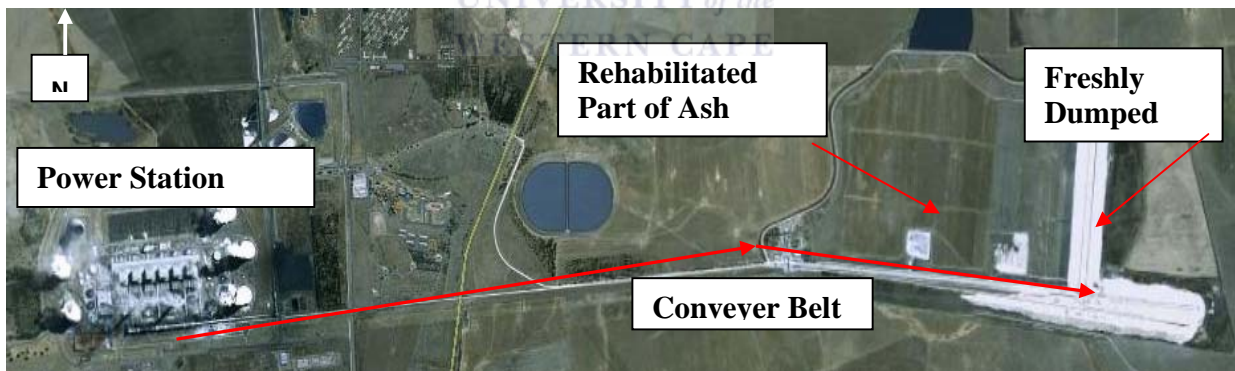
Figure 3.1 Aerial view of the Tutuka Ash dump, ash transported via conveyer belt to the ash dump. Rehabilitated parts of the ash dump can be observed and also freshly dumped ash.
