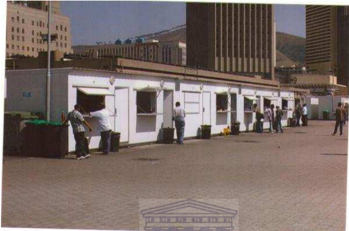
Figure 11: The new kiosks built for informal traders on the Station Deck in Cape Town ( Photograph F. E. Tabe)
