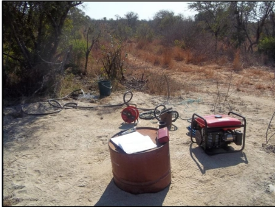
Figure 4.11 Equipment used during a pump test.
