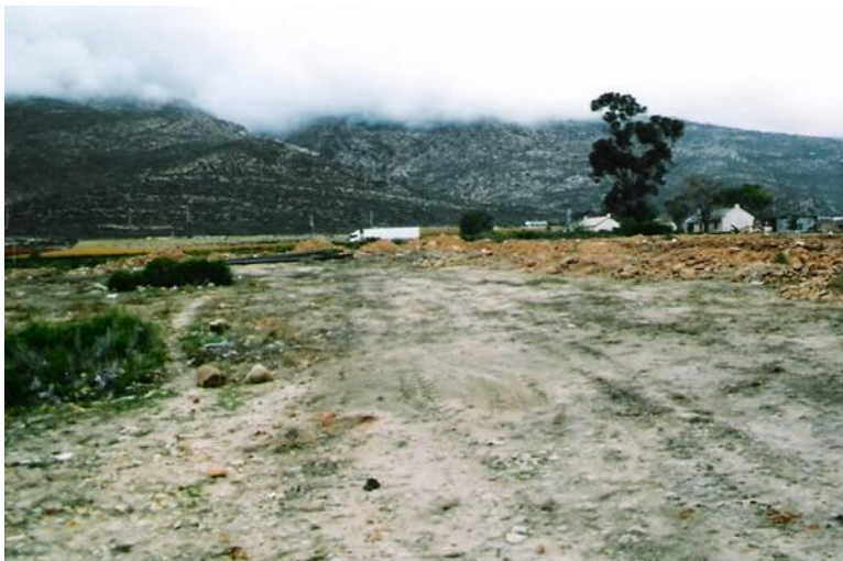
Figure 2.14: The same natural habitat of G. multifolia and G. villosa being destroyed for the laying of sewerage pipes. (photo taken in 2006).
