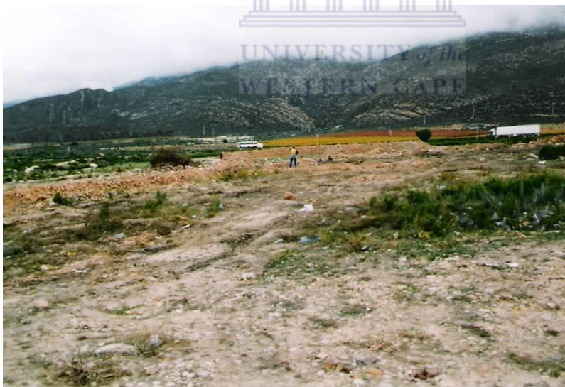
Figure 2.16: The same section under construction for the laying of more sewerage pipes (photo taken in 2006).
