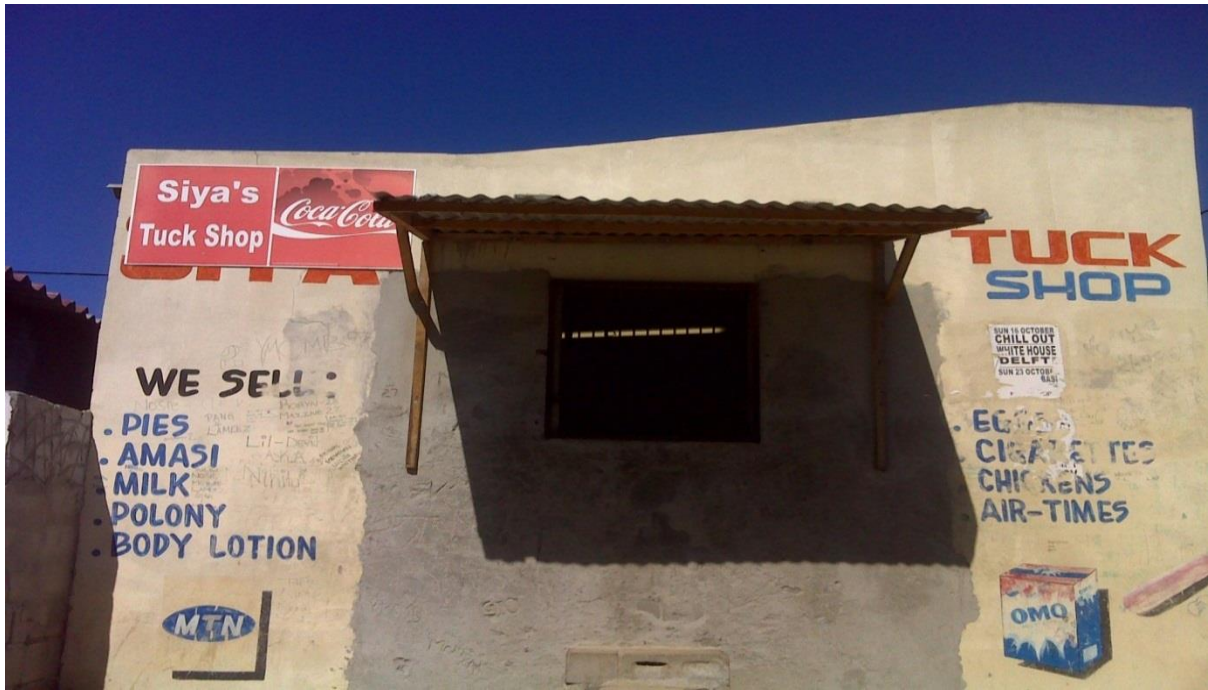
Figure9: This building used to be a free standing garage, now a Somali spaza shop.
