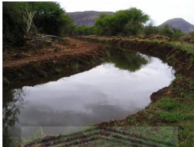
FIGURE 16 HEREFORD: UNLINED SECTION OF HEREFORD CANAL, 2004
