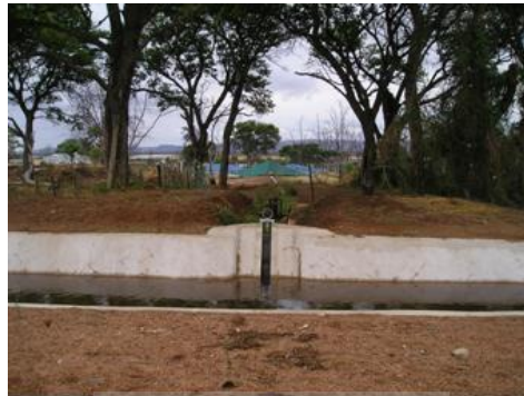
FIGURE 14 HEREFORD: ABSTRACTION POINT AND CANVAS-PROTECTED TANKS FOR TEMPORARY SUPPLY OF RAW WATER FOR DOMESTIC USE, 2004
